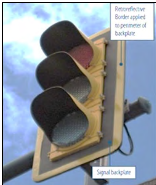
Figure 32: Backplate with a retroreflective border (Source: FHWA)
