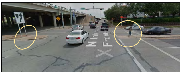
Figure 28: One-stage pedestrian median refuges in Austin TX. (Source: Google Maps)
