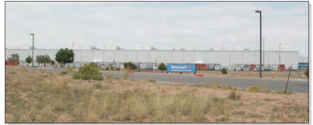
Commercial development west of I-25
