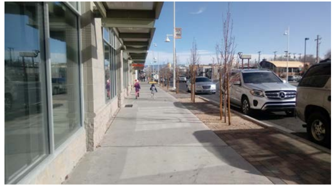
New wider sidewalks and pedestrian scale lighting on Central Avenue in Nob Hill added during ART construction
