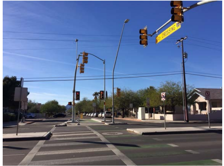
HAWK signal with median refuge for pedestrians and bicyclists in Tucson, AZ
