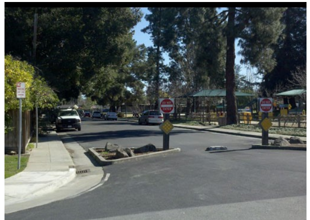
Street Closure near Park in Palo Alto, CA. Source: NACTO Urban Bikeway Design Guide
