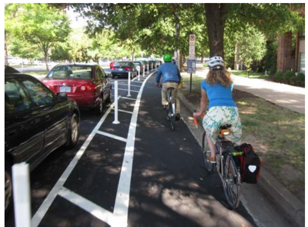
Protected Bike Lane in Arlington, VA. Source: City of Arlington
