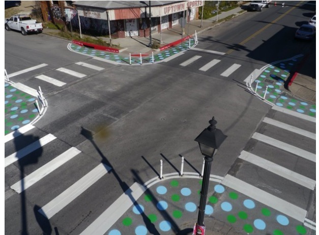
Curb extension in Austin, TX. Source: City of Austin
