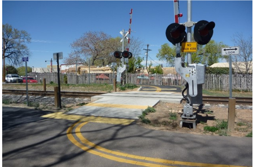
Acequia Trail crossing in Santa Fe Source: Rio Metro
