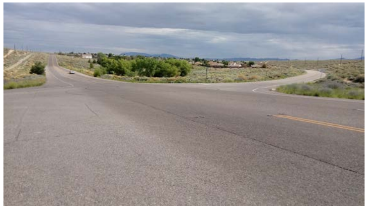
Rural Valencia County (Rumble strips on hill approach)
