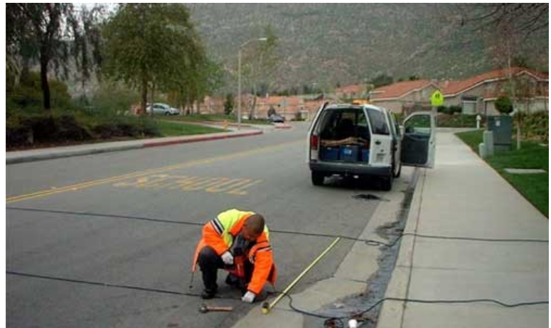
Setting up Traffic Count Tubes Source: City of Moreno Valley
